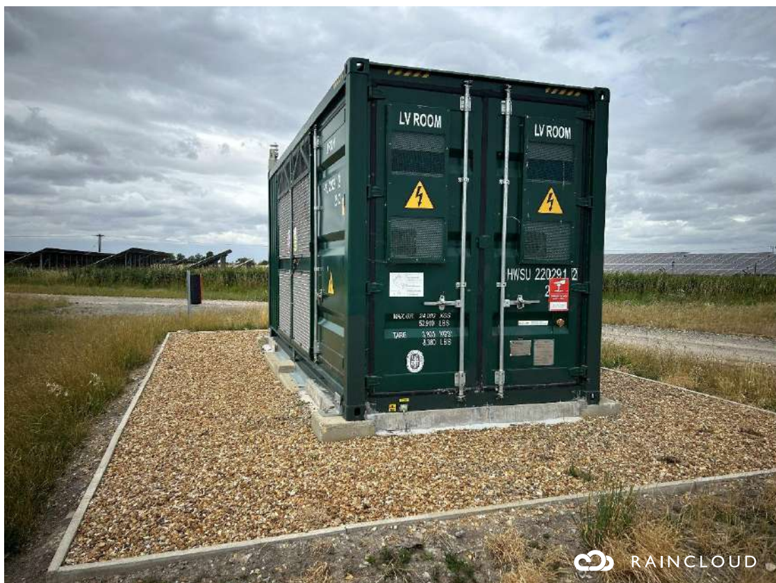
Plate 12-33 Conversion unit gravel surround
